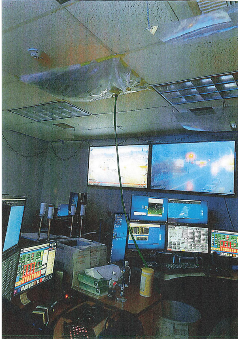
Water leaking through the ceiling of the 911 Dispatch Center is being diverted into garbage cans to avoid the computer equipment.
