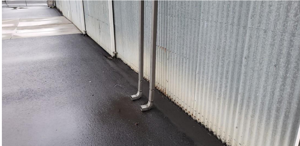
Pavement and Gutters Installed; Photo: Jury Member
